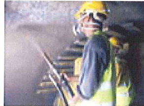
The nozzleman applies a novel type of near-zero rebound shotcrete directly behind the cutterhead support of the excavating Robbins TBM
