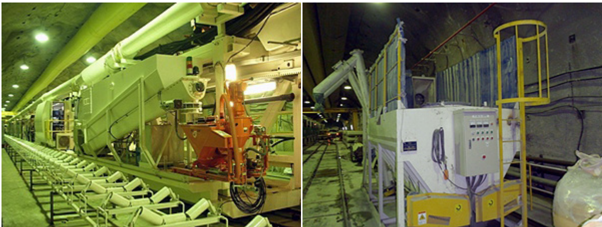
Figure 2. The fiber mortar system installed on TBM & the loading station at the bottom of the adit
