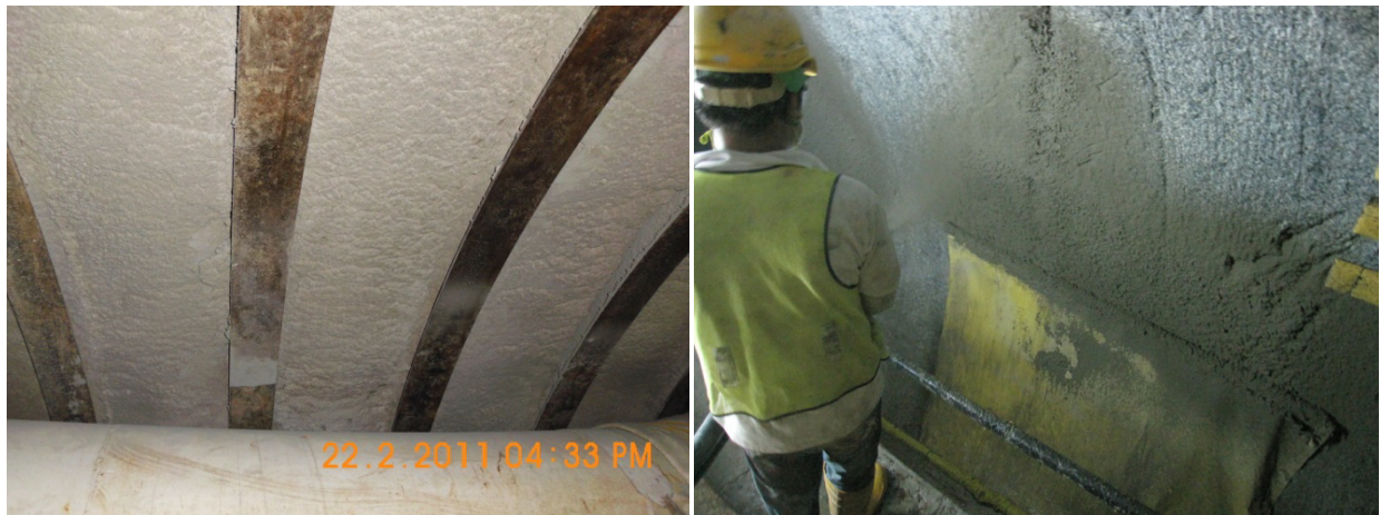
Figure 3. The fiber mortar system applied with ring beams (left) and one man application (right)
