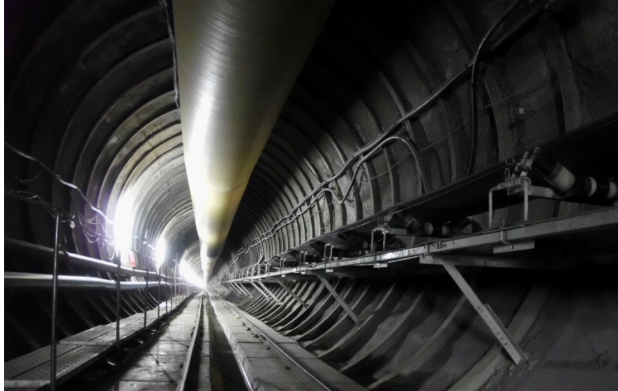
Figure 4. A section of completed tunnel looking outbye (away from the machine) in poorer ground conditions with ring beams and fiber mortar completed. Note the continuous conveyor to the left of the photo and segment installation in the invert.
