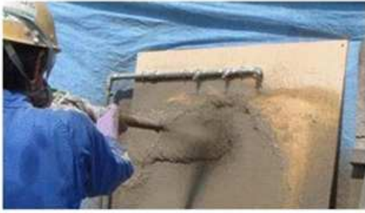
<Spraying under water inflow>
